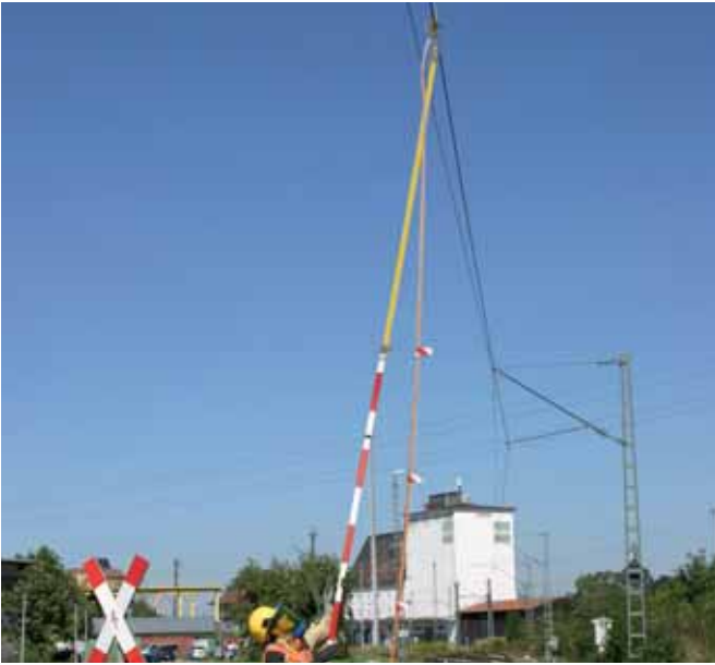
Attaching a railway earthing device.
