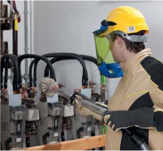
Live cleaning of a transformer using the TRS MS dry cleaning kit
