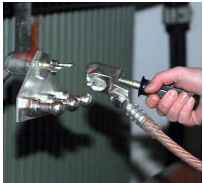
Earth connecting plate with fixed ball points and ball head cap with plastic handle
