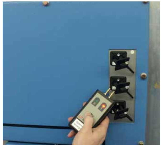
Self-test of a DEHNcap/A voltage indicator
