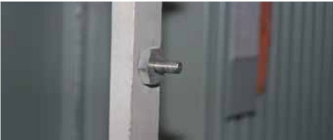
Bolted-type earth connector with M12 threaded pin on an earthed part of an installation.
