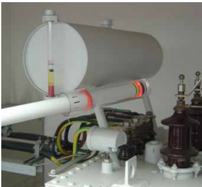
HSA 205 high-voltage indicator with insulating cap used on a switchgear installation.
