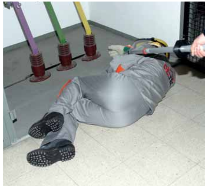
Insulated RST rescue rod used to rescue an electrified victim from the live working zone
