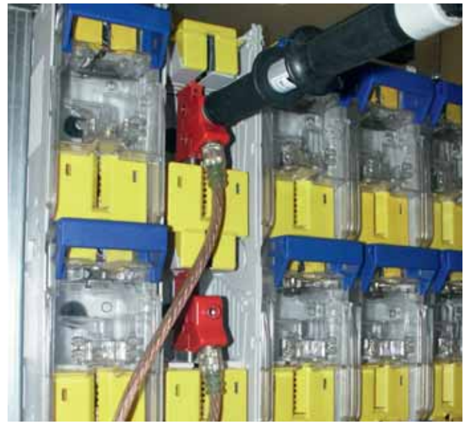
Attaching a fully insulated earthing and short-circuiting device using an earthing handle of type VI
