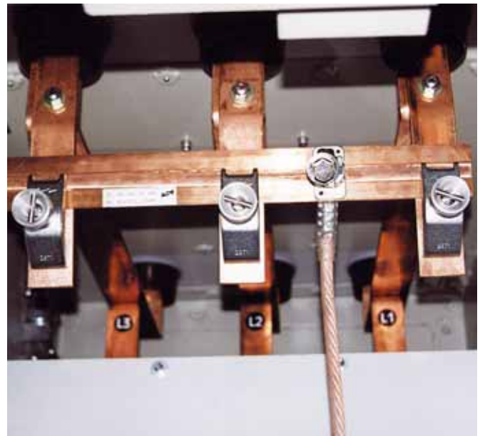
Short-circuiting bar with earthing cable on a switchgear installation
