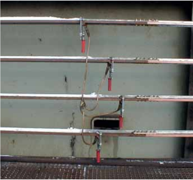
Three-pole earthing and short-circuiting device with screw clamps.
