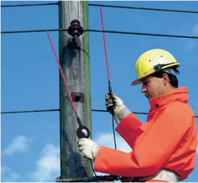
Two-pole SPN voltage detector used with extension prods for overhead lines
