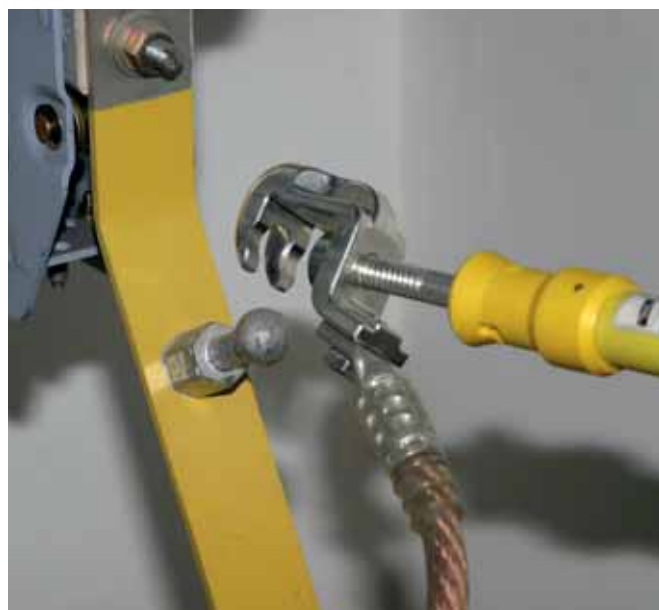
Connecting the phase cable end with universal clamp to a fixed ball point
