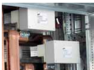
Short-circuiter above the supply switch
